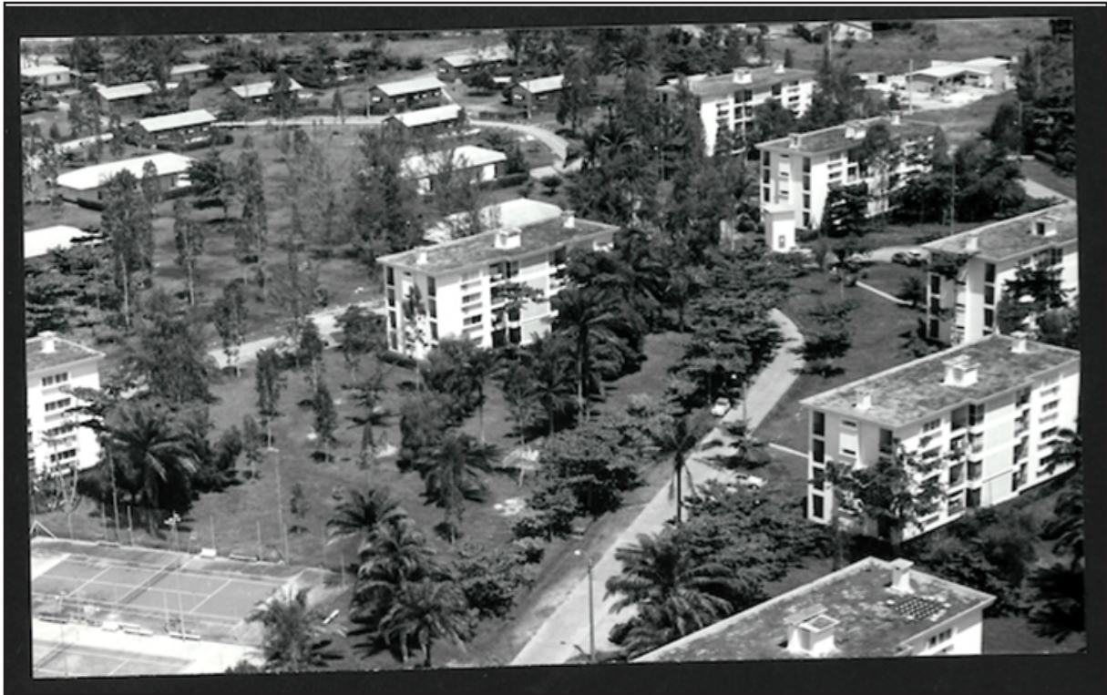
FIGURE 2: ELF-SPAPE APARTMENT COMPLEX FOR ITS EXPATRIATE WORKERS.
