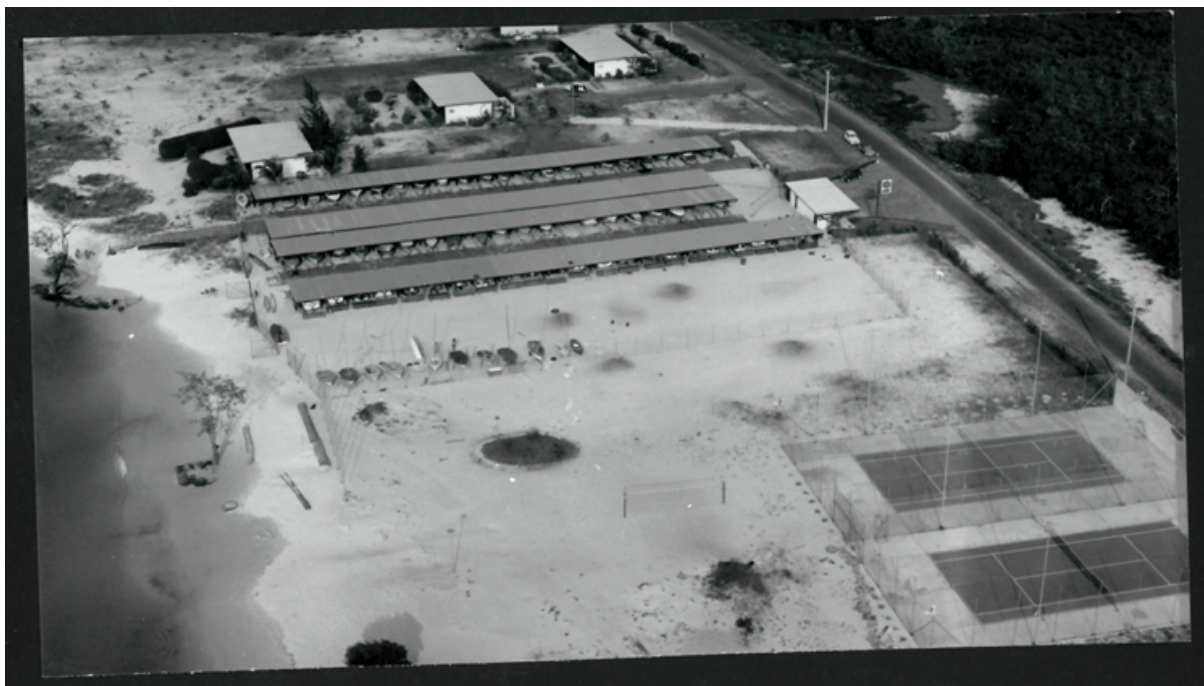
FIG. 3. CLUB SOGARA BUILT ALONGSIDE THE HOUSING COMPLEX DESTINED TO HOST THE REFINERY'S EXPATRIATE WORKERS.
